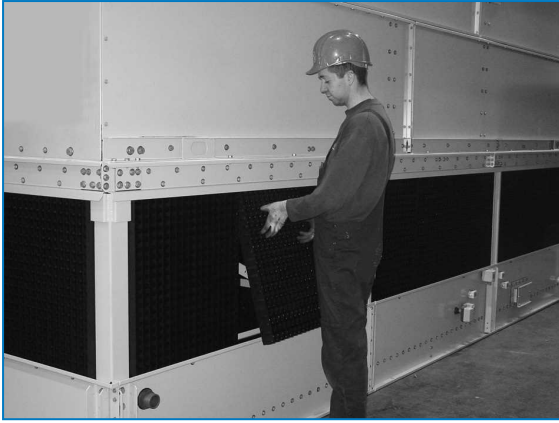
Remove combined inlet shields
