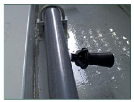
A sump sweeper piping system **increases water circulation and agitation** in the basin and is designed to be used in combination with a <u>filtration</u> system. It does all this:
