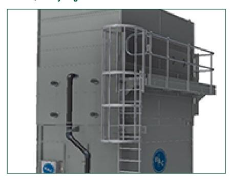
A ladder, safety cage and handrails are all installed for easy access to the unit top and easier and safer inspection and maintenance, in line with EU safety directives.
