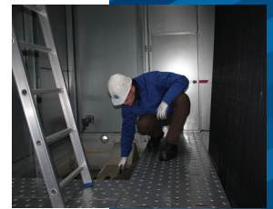
BACross® fill guides the water down
