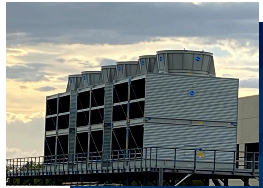
S3000E open cooling towers
