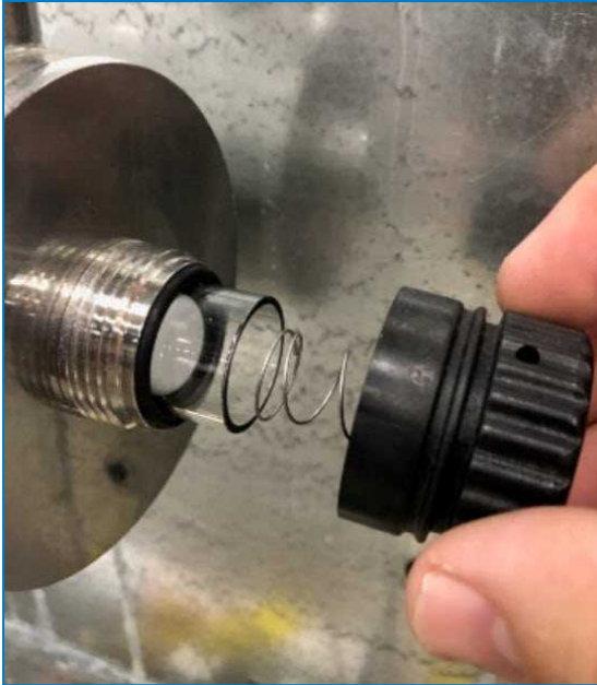
UV quartz sleeve removal
