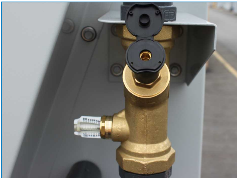
Water flow adjustment screw
