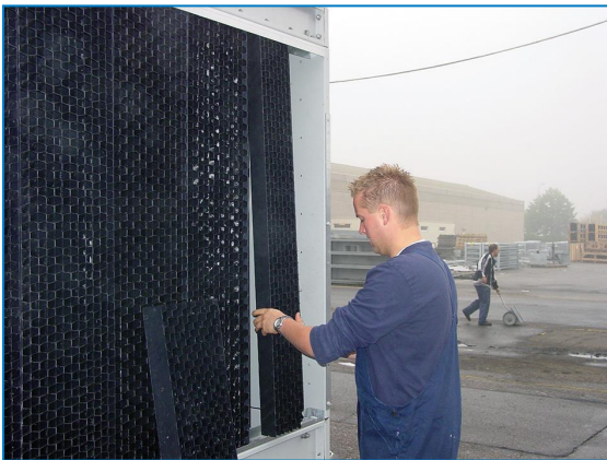
Remove combined inlet shields
