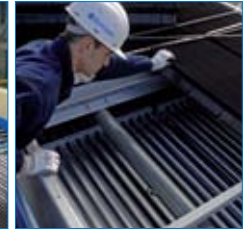
on site services
