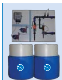
Correctly sized chemical drums and bunds
