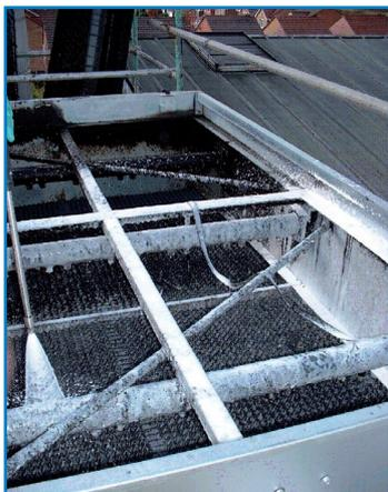
Keeping surfaces clean within a cooling tower or evaporative condenser system not only ensures that the thermal performance is optimised but also that the growth of biofilm and harmful bacteria, including legionella, is avoided. This is achieved by effective water treatment and a programme of manual cleaning and disinfection.
