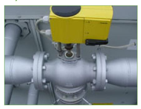
The **3-way-valve** is an control arrangement which:
