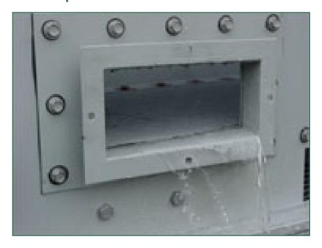
A factory-installed clean out port
